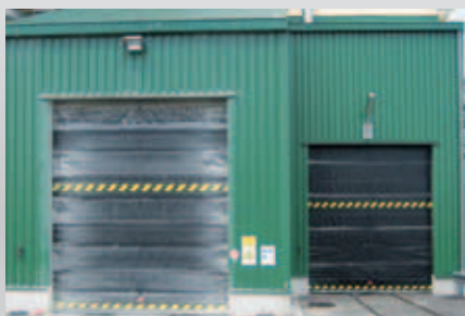
High speed door in Atex area (dust).
