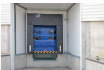
High speed door in loading bay.
