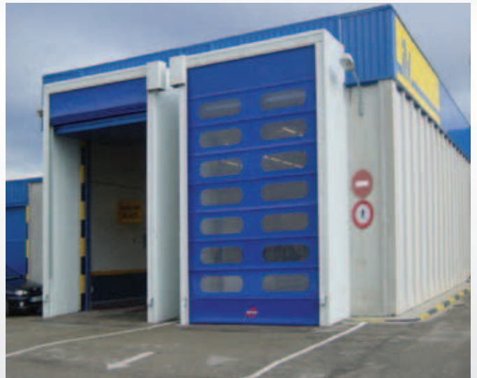
High speed doors with side and upper enclosures installed on the outside.
