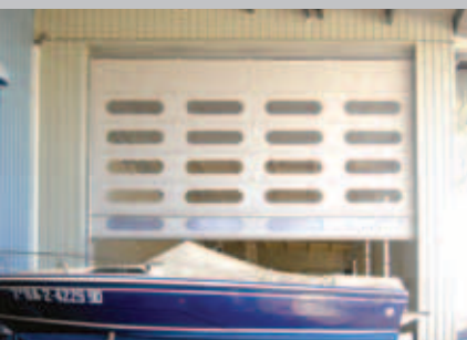
High speed door in a cabin.
