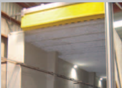
High speed door in a cabin.
