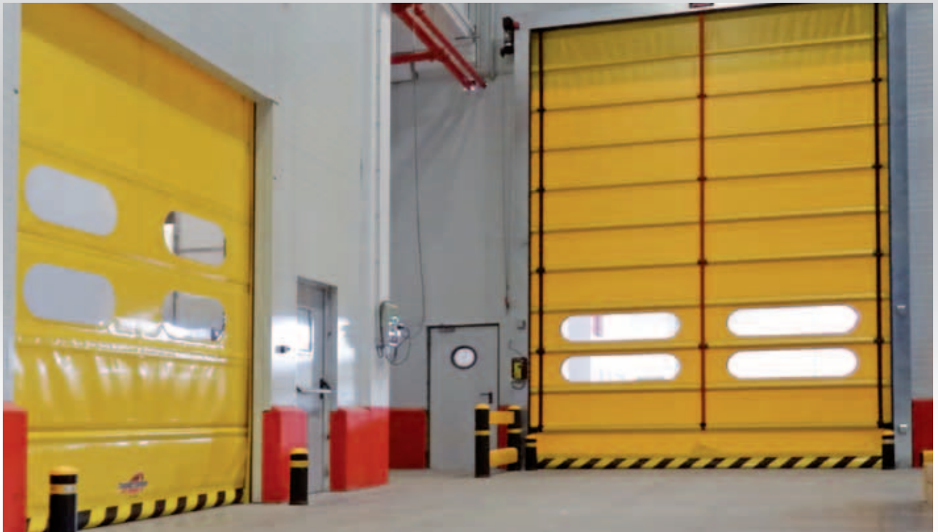
Instant Pass® BASIC at logistic warehouse.
