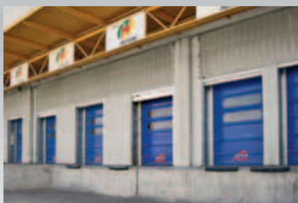
High speed door in loading bays.
