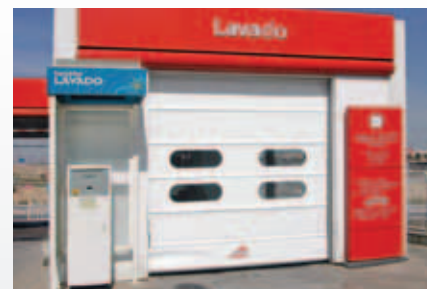
High speed door, car wash.
